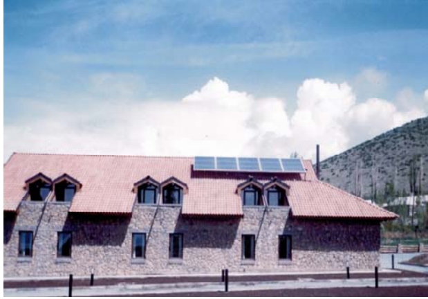
Figure 13. Solar Water Heating System, Hotel Blue Sevan
