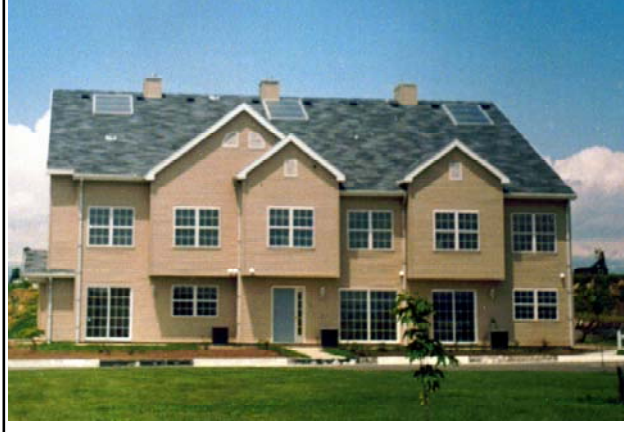
Figure 14. Solar Water Heating System, Private house, Vahakni Community, Yerevan
